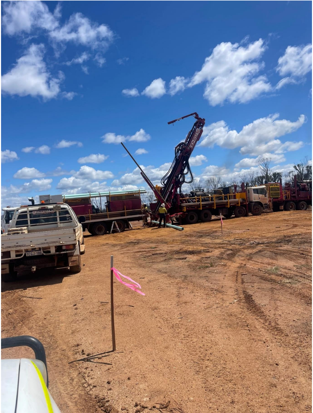
Figure 3: Extensional RC Drilling at Kat Gap
