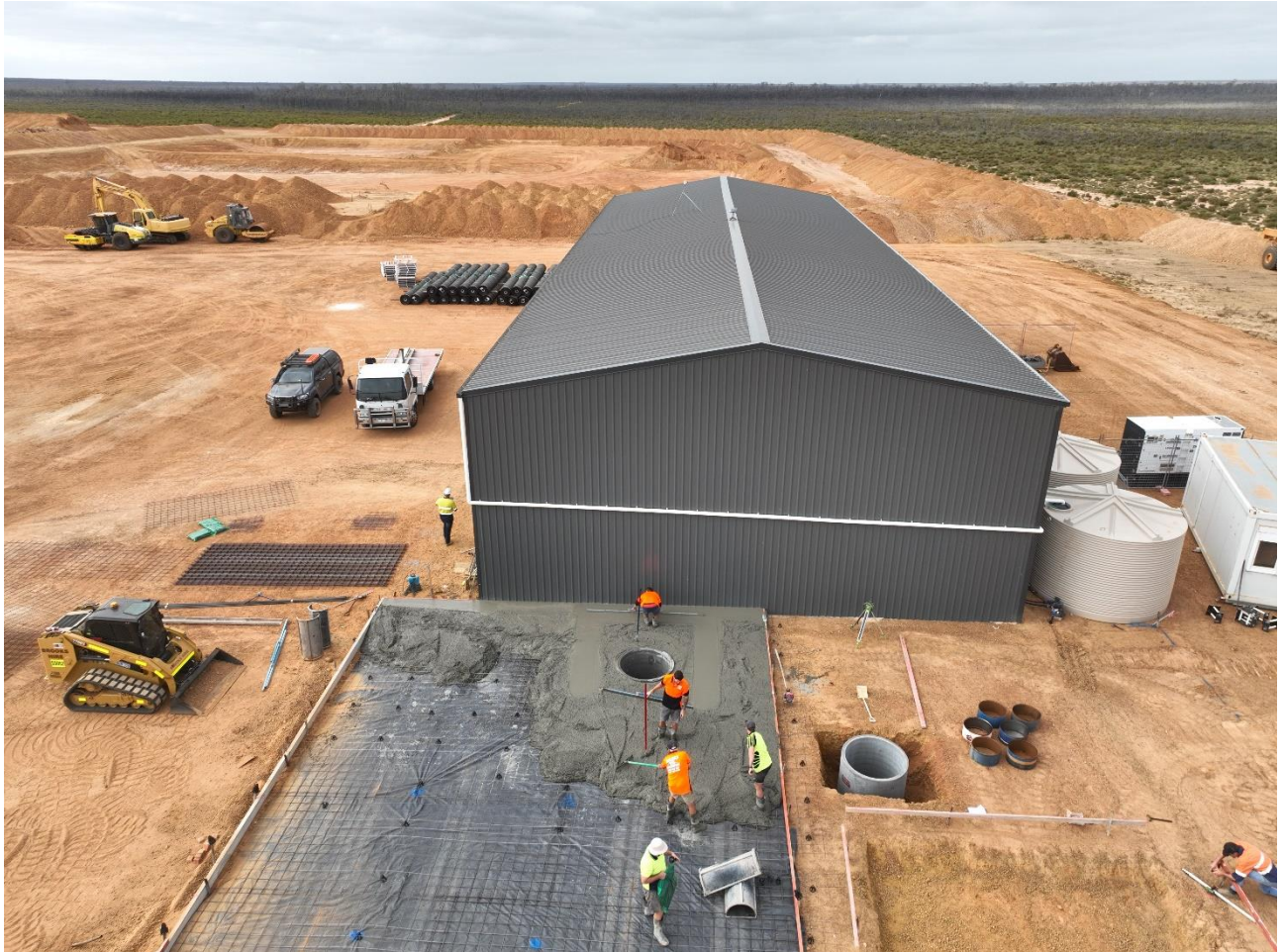
Figure 3 & 4: Foundation outside the shed with sumps.
