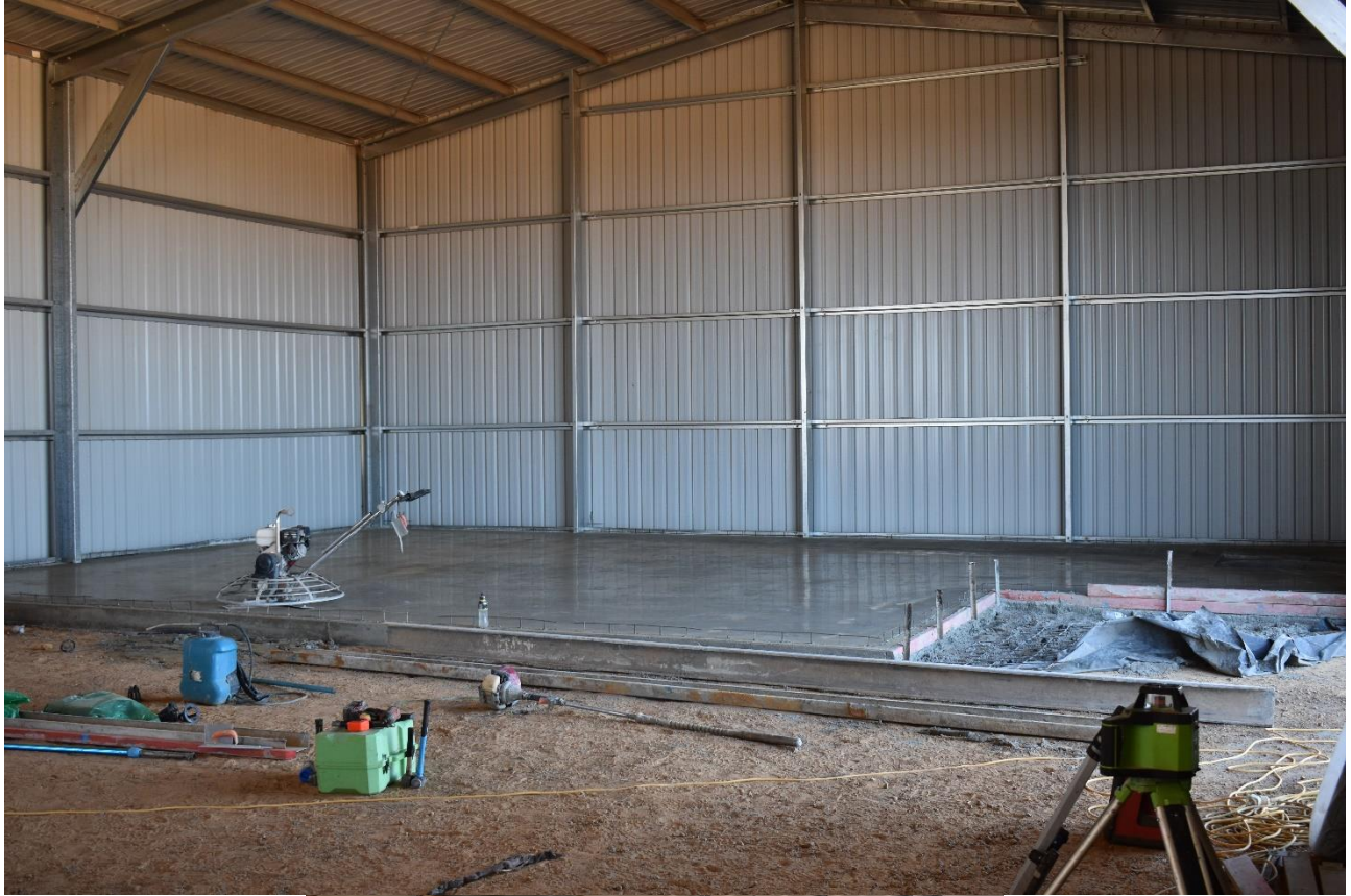
Figure 3 & 4: Foundation inside the shed for Gold Room.
