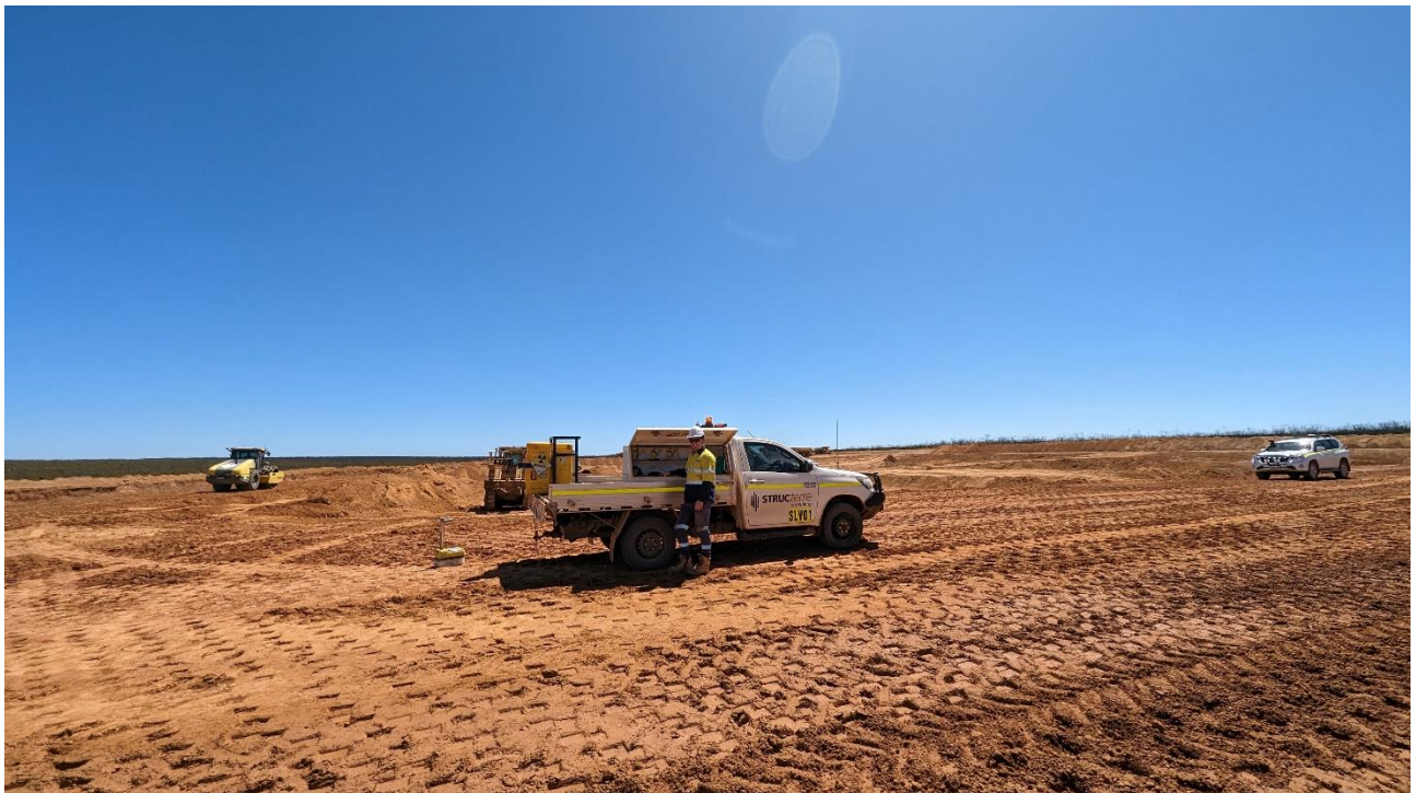
Figure 2: REC Consultants managing construction of TSF.
