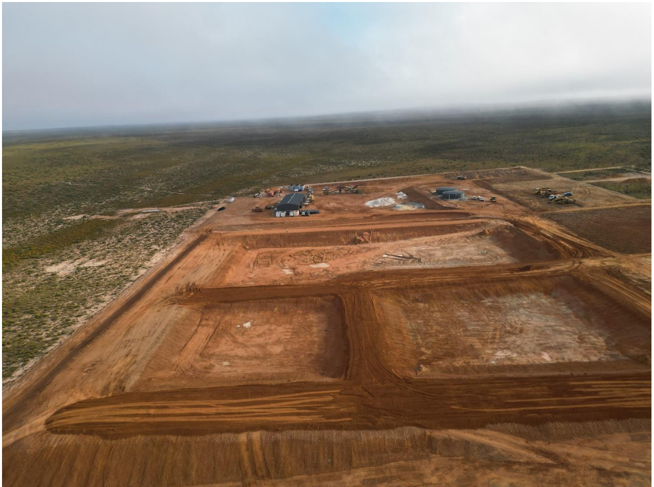
Figure 1: Kat Gap Processing Facility showing TSF progress.
