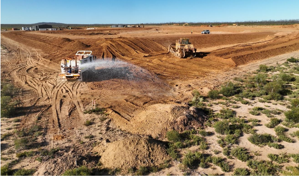
Figure 3 & 4: Machines working on TSF & Aerial view of Kat Gap Processing Facility.
