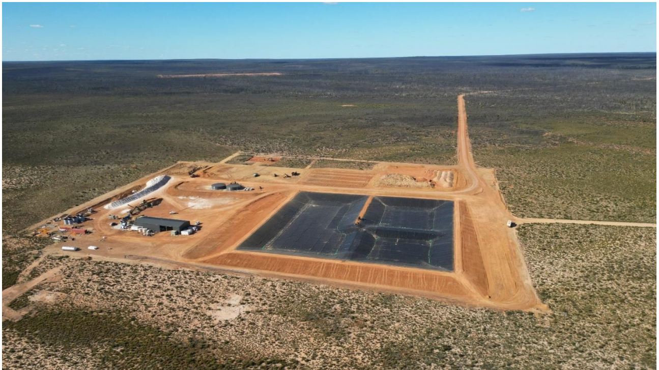
Figure 1: TSF HDPE lining works 100% complete.
