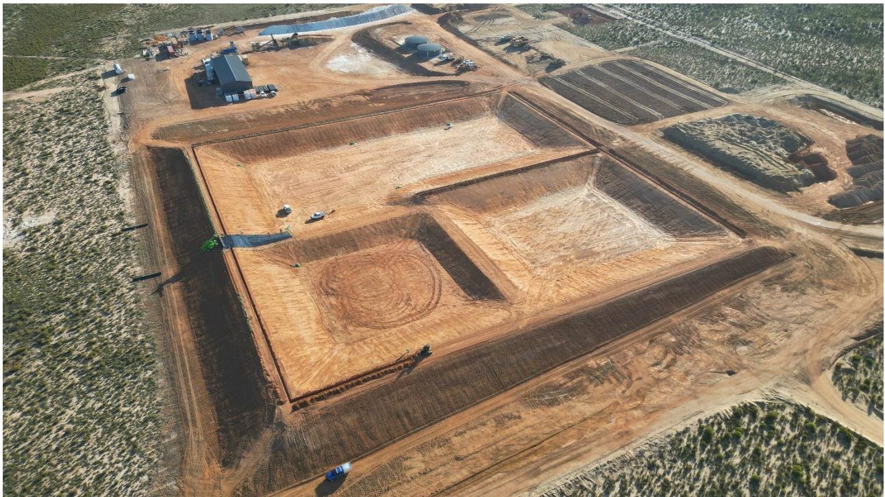
Figure 2: Commencement of Kat Gap dam lining.
