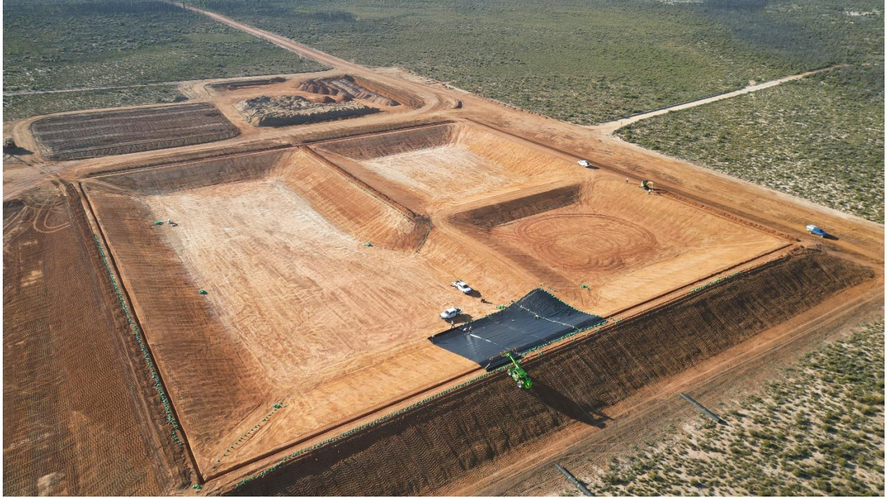
Figure 3: Kat Gap Dam lining in progress.
