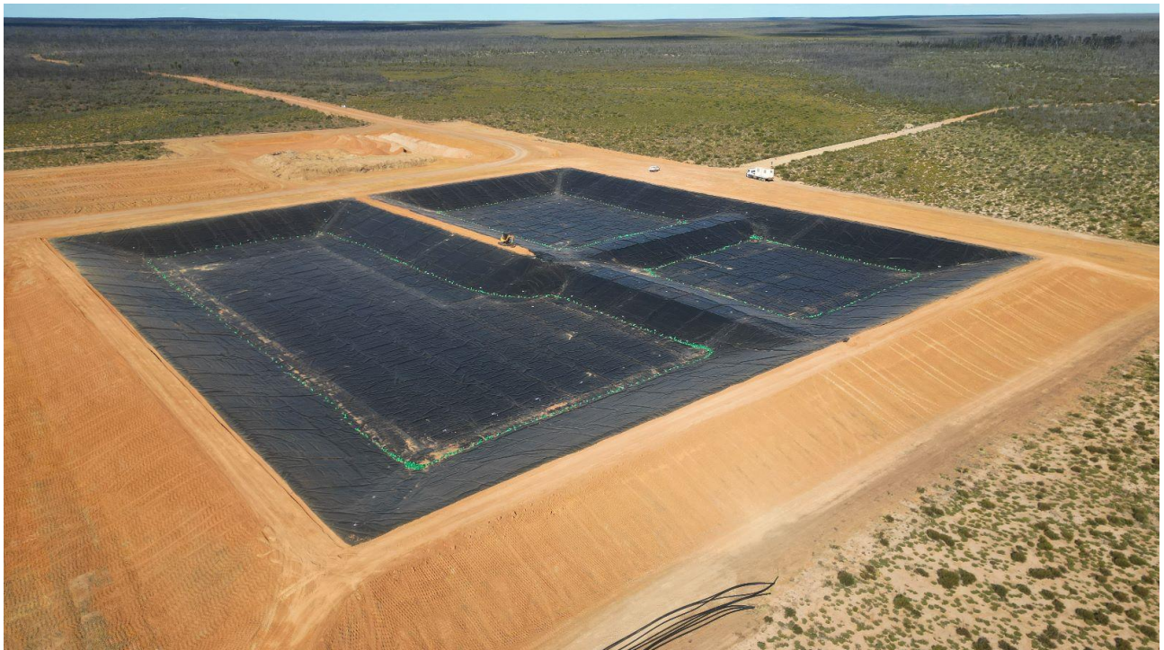
Figure 4: Kat Gap dam lining completed.
