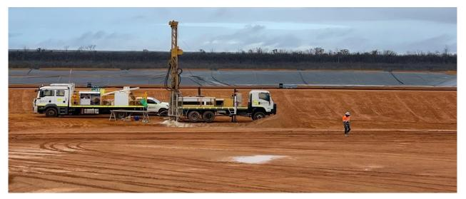
Figure 2 TSF Piezometer Installation And Drilling
