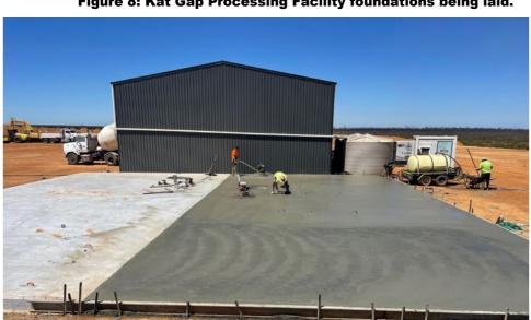
Figure 8: Kat Gap Processing Facility foundations being laid.
