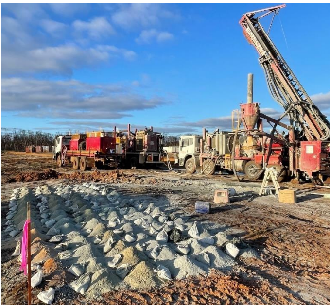
Figures 1 & 2: Drilling at Kat Gap
