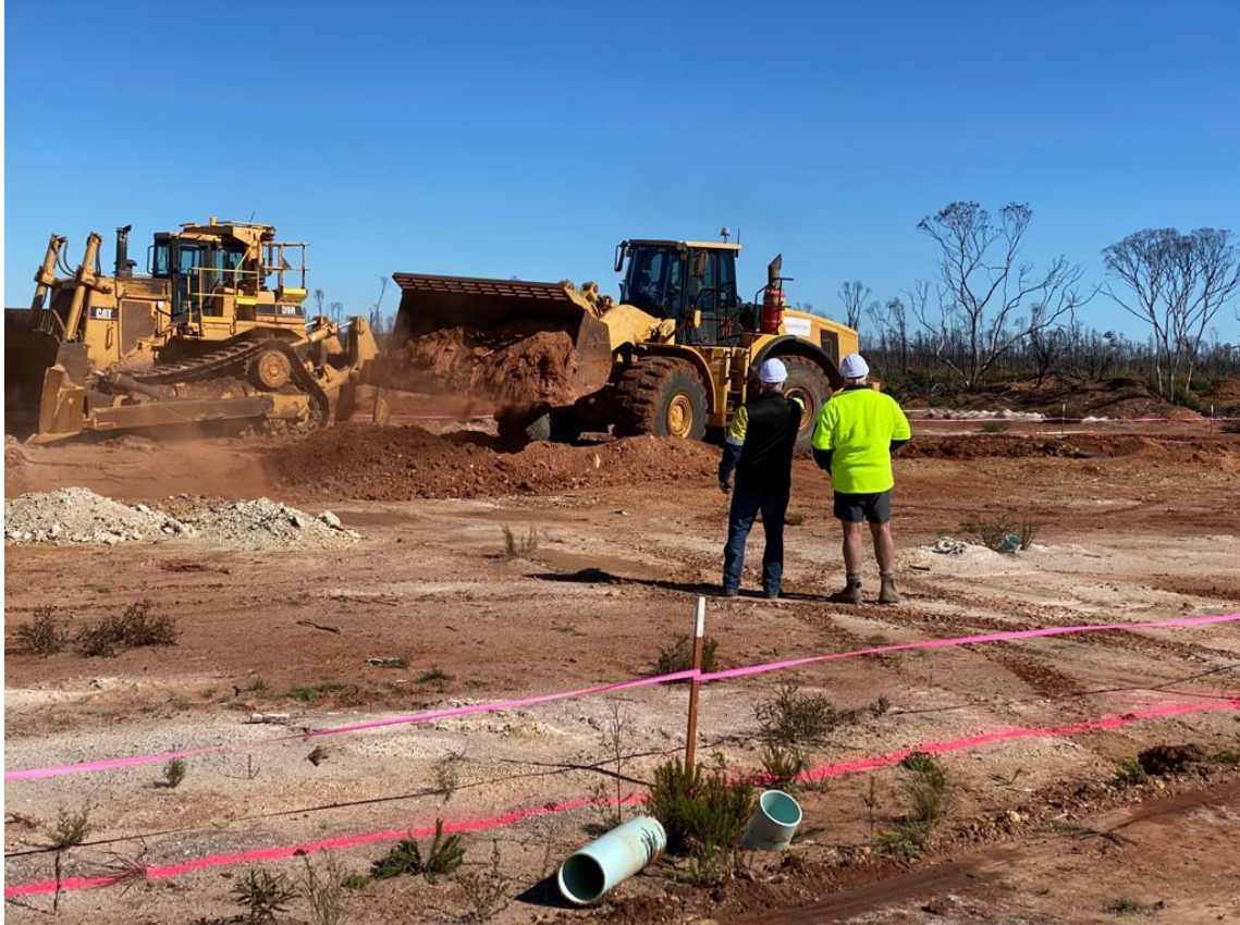
Figure 4: Dozer and Loader commence pushing back topsoil at Bulk Sample Pit, Kat Gap.
