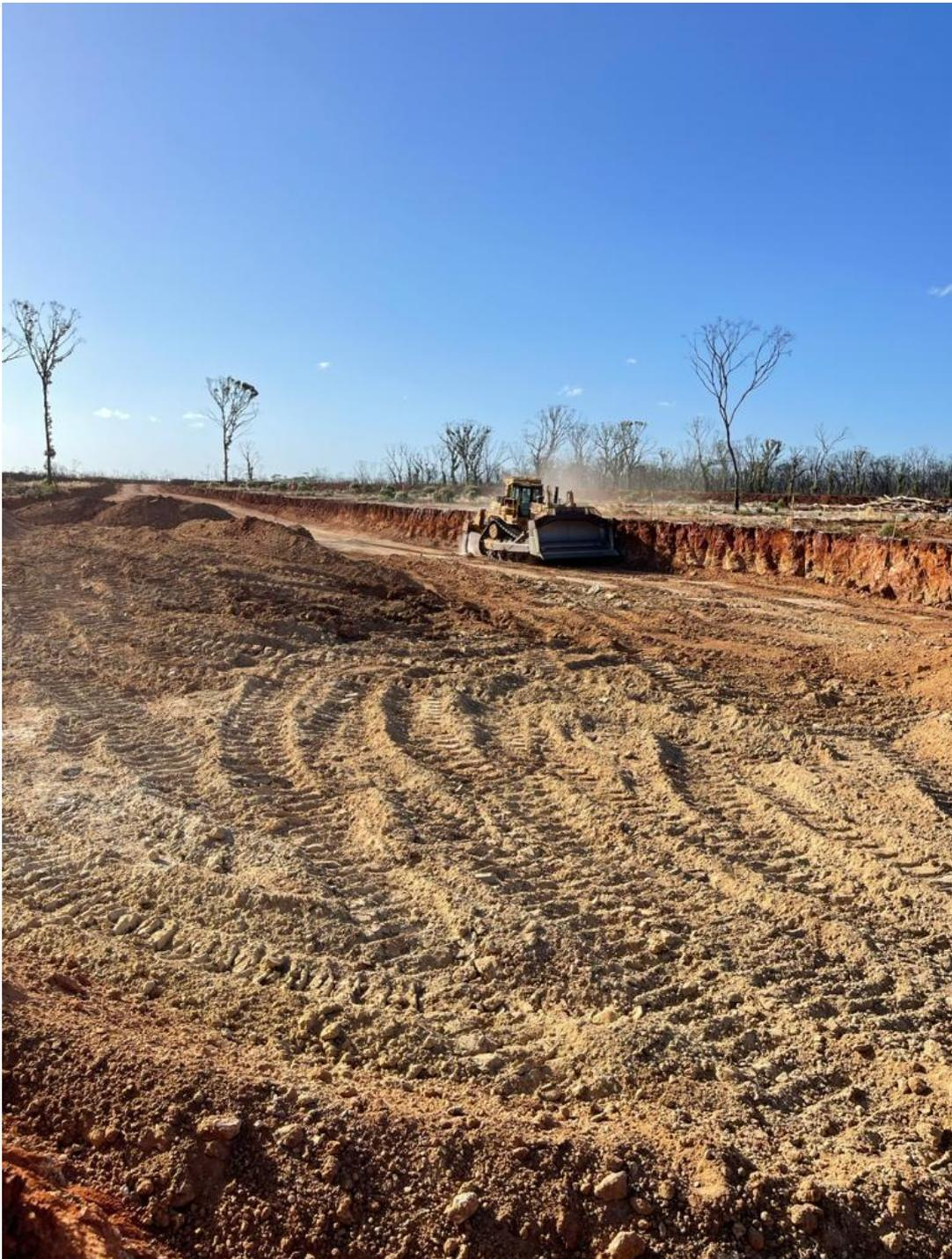
**Figure 5: D9 Bulldozer ripping overburden in pit**
