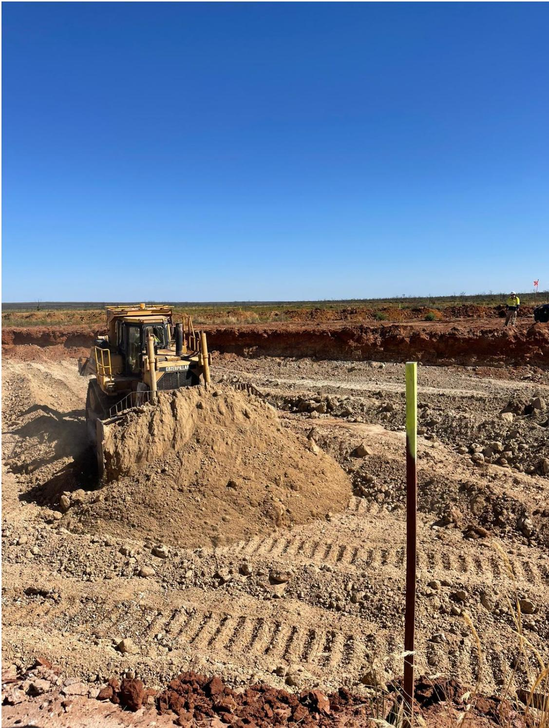
**Figure 7: Dozer pushing overburden in the Bulk Sample Pit.**
