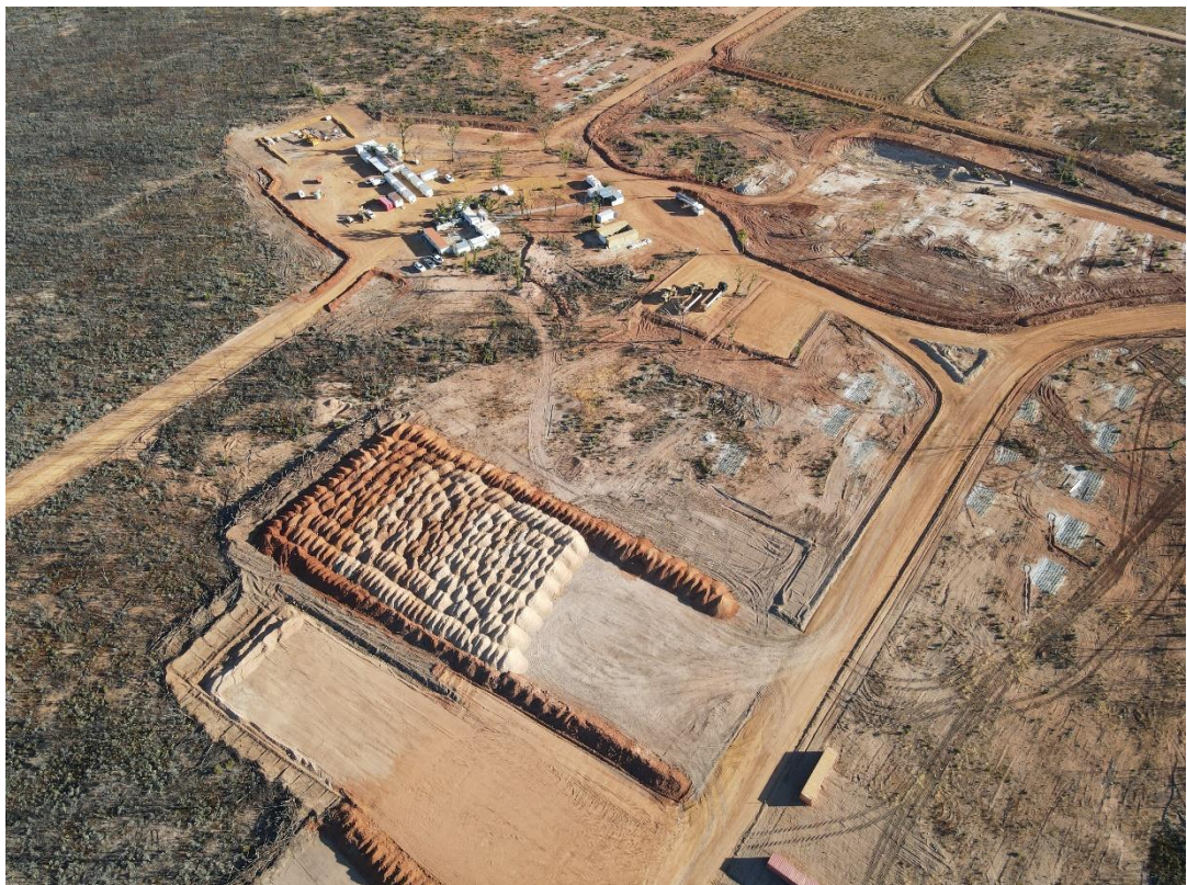
Figure 1: Kat Gap – Looking Northwest.
