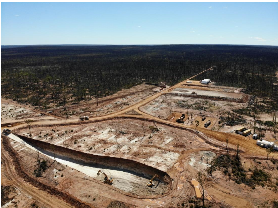
Figure 6: Aerial view of Bulk Sample Mining Pit
