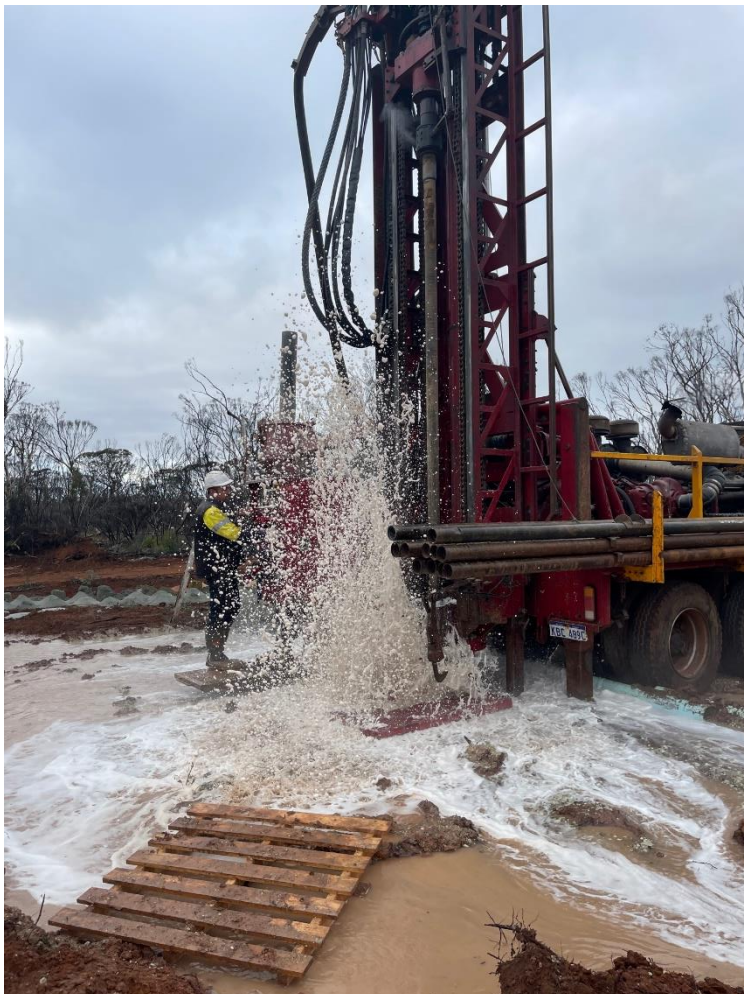
Figure 1: Photo of water bore GPLWB001 being drilled
