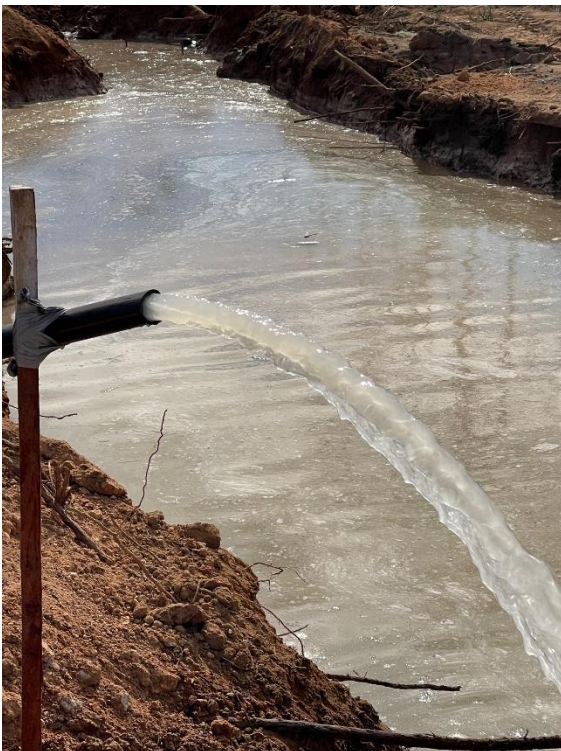
Figure 2: Photo of water bore GPLWB001 being drilled and water from bore.
