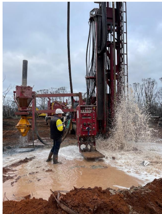
Figure 2: Photo of water bore GPLWB001 being drilled and water from bore.
