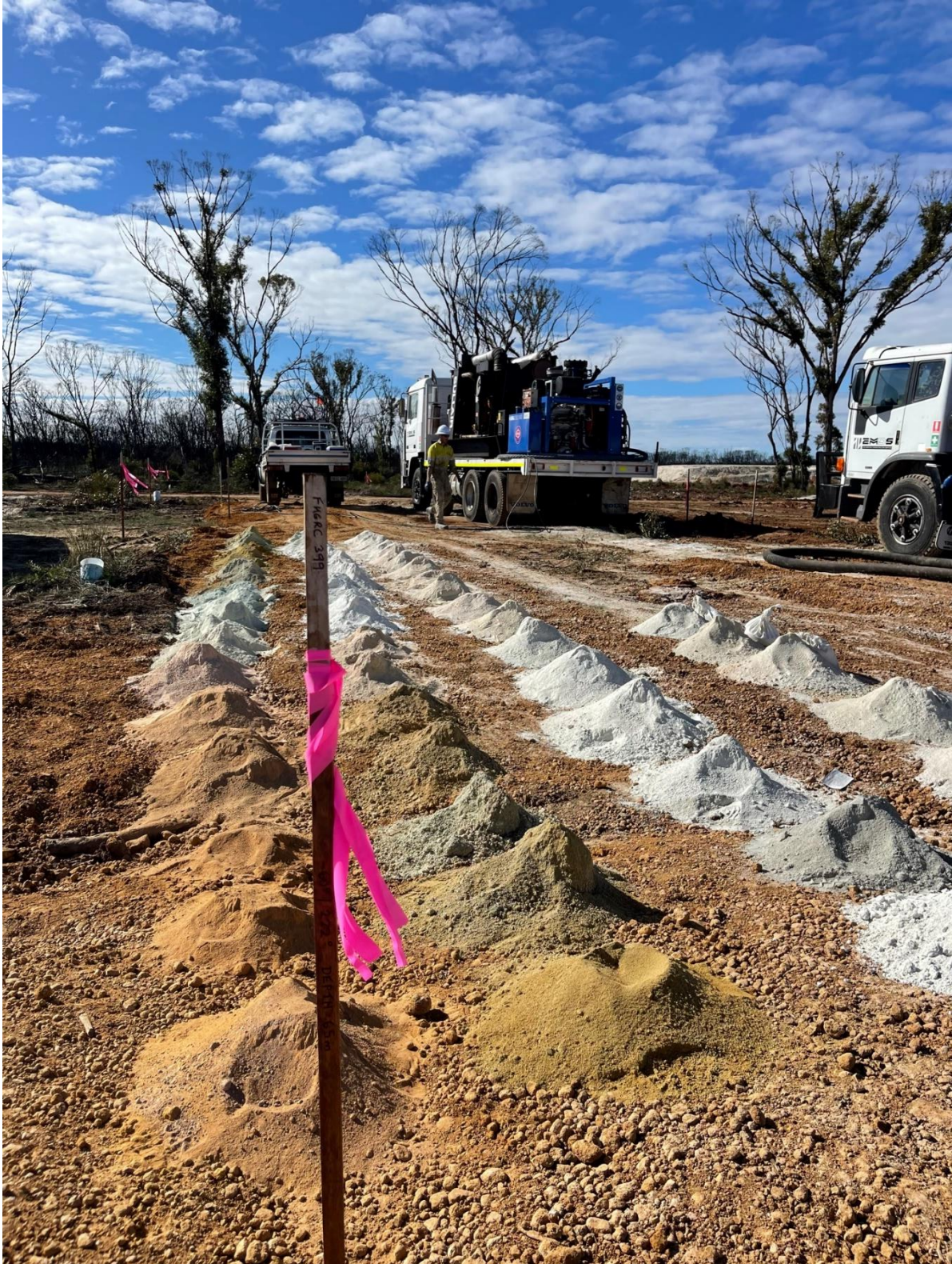
Figure 2: Drilling at Kat Gap
