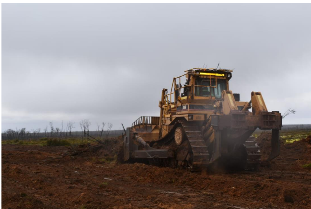
Figure 2: Bulldozer clearing at Kat Gap site.
