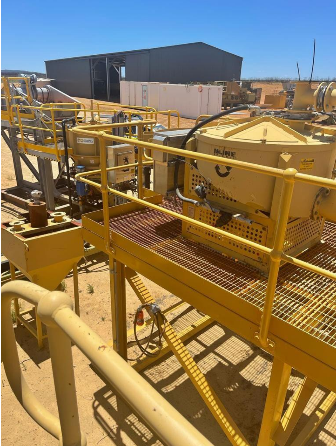
FIGURE 2: Gekko plant components ready for construction at KAT GAP
