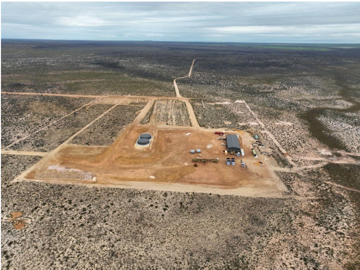
FIGURE 4: Aerial view of Kat Gap Processing Site
