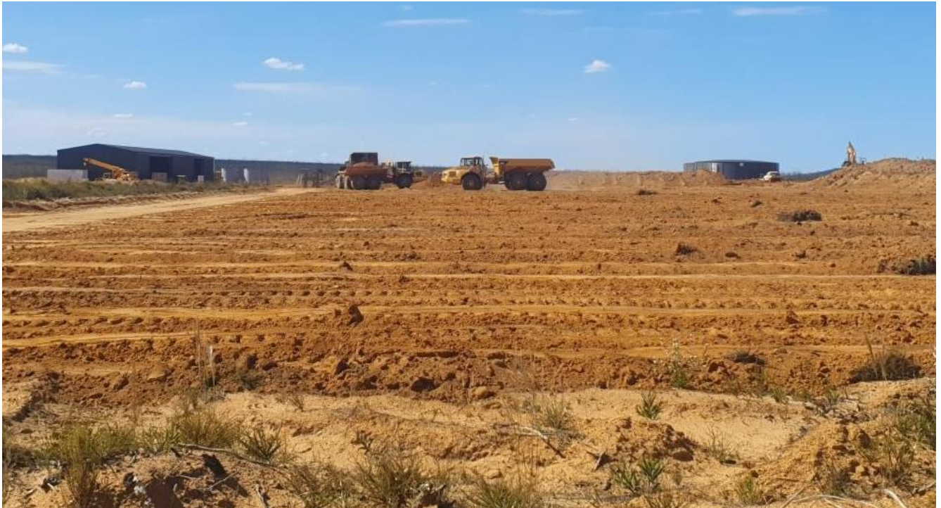
Figure 1 & 2: TSF area being cleared
