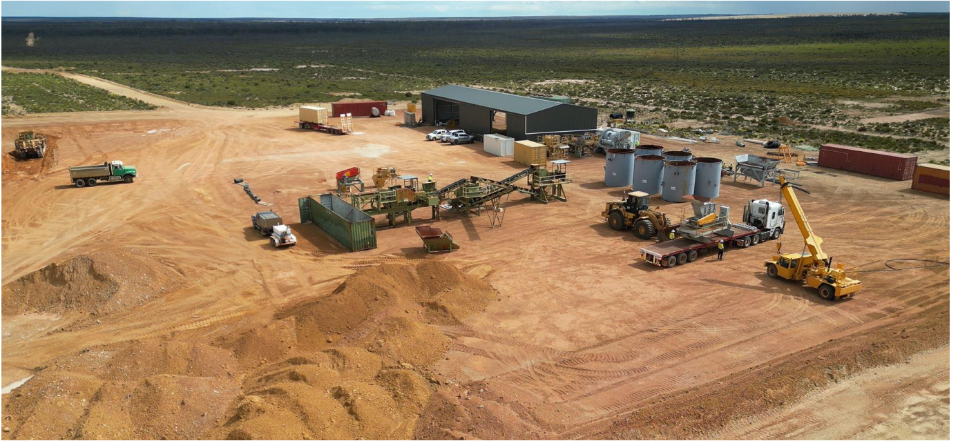
Figure 3 & 4: Plant being assembled and water storage tanks
