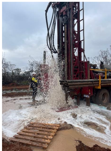
Figure 4: Photo of water bore GPLWB001 being drilled and water from bore. 1
