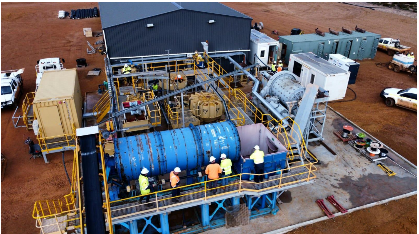
Figure 1 – Kat Gap Gold Processing Plant.
