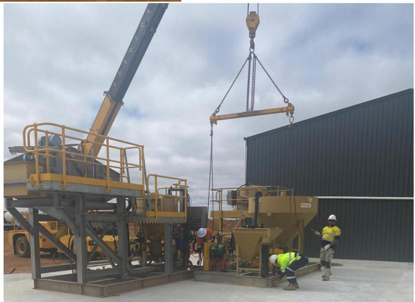
**Figure 9: Ball mill being placed on foundation.**
